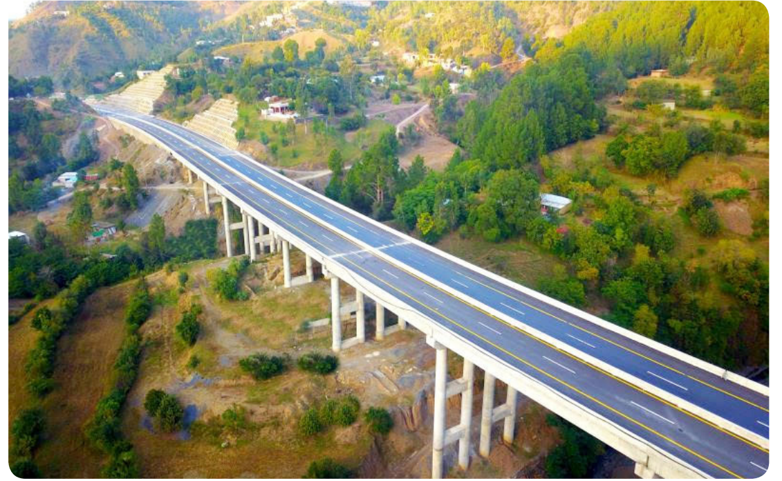
ISLAMABAD: A view of CPEC highway Havelian Thakot section which has been completed. - DNA
