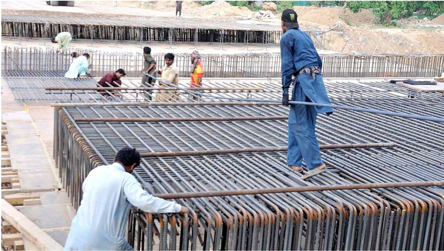
ISLAMABAD: Workers busy in construction of underpass on Faisal Avenue. - APP
