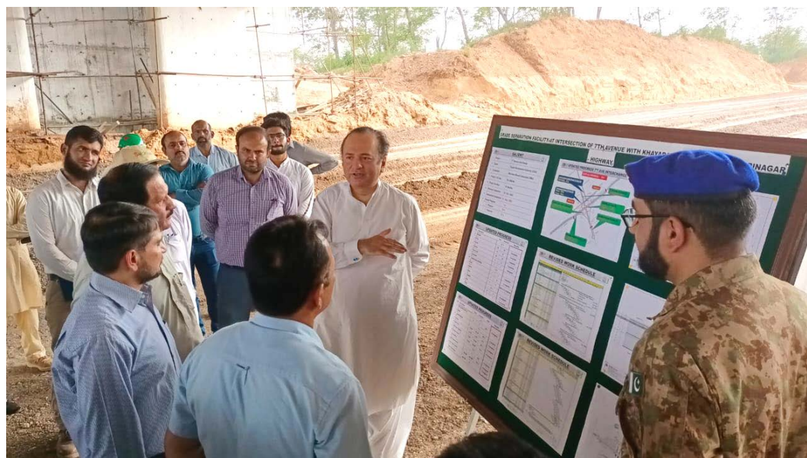
ISLAMABAD: Chairman of CDA on visited the ongoing construction work at Seventh Avenue Interchange and Rawal Dam Chowk. Officers of the Engineering Wing were also present on the occasion. - DNA
