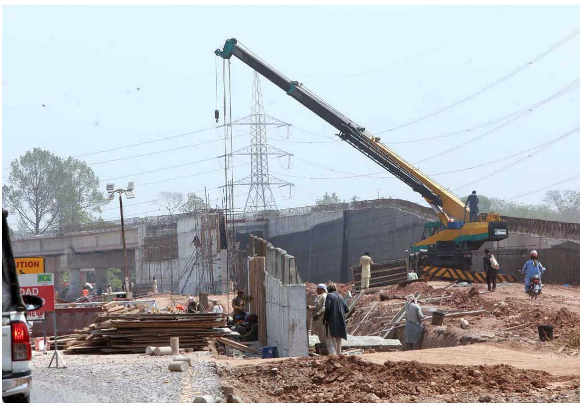
ISLAMABAD: Heavy machinery is being used at the site of a flyover at Rawal Dam Chowk. — APP
