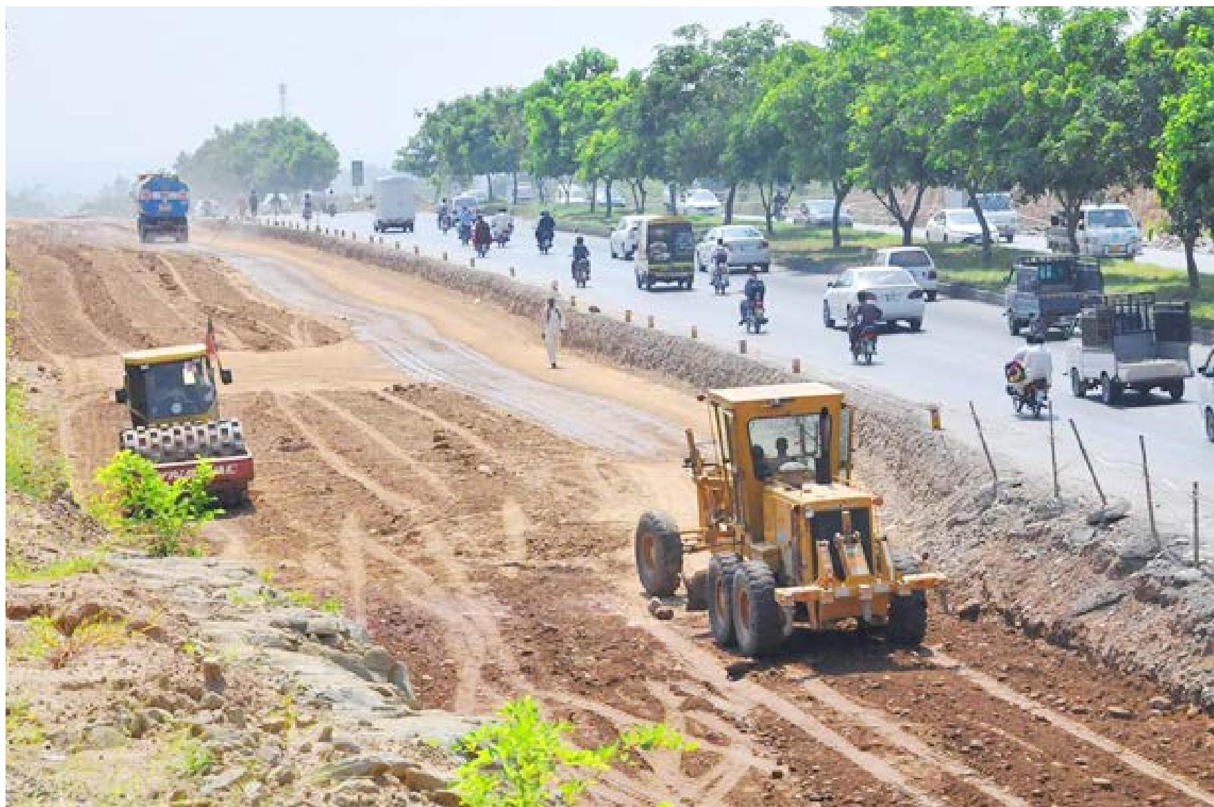
ISLAMABAD: Heavy machinery being used in construction work of Islamabad Expressway during development work in the city. - APP
