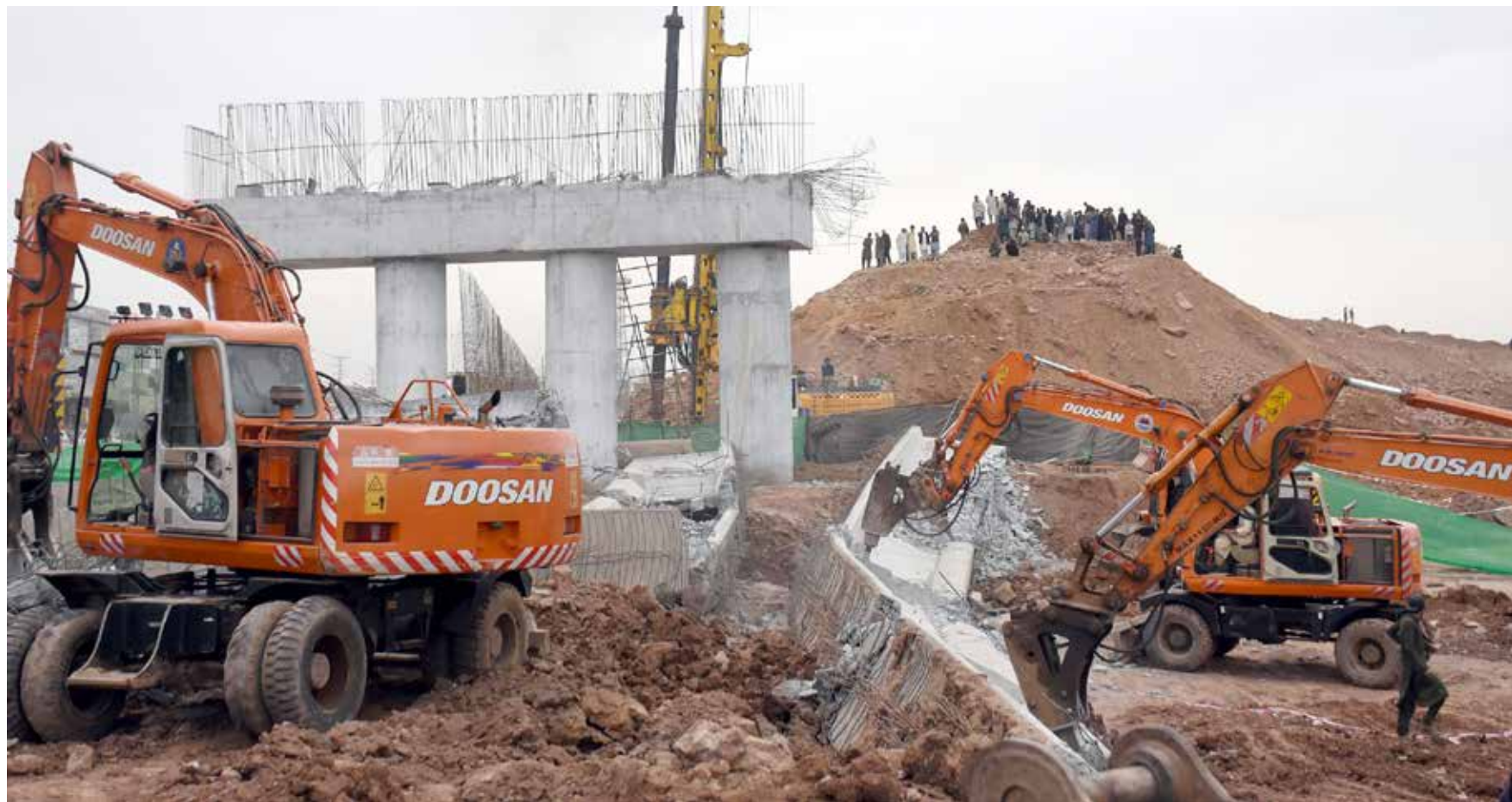
ISLAMABAD: Workers are busy removing debris after the collapse new contracted Bhara Kahu enter change flay over bridge pillar with the help of heavy machinery, in Federal Capital. -Online
