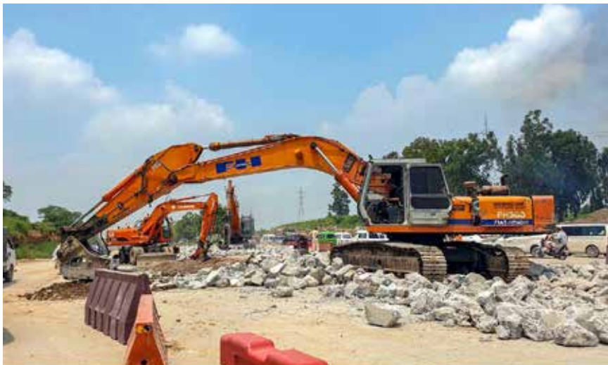
ISLAMABAD: Heavy machinery being used to expand lanes on Islamabad Expressway.—APP
