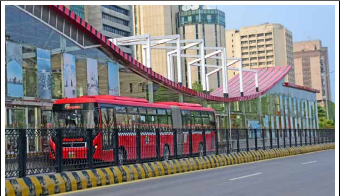
ISLAMABAD: The Metro Bus Service, which was shut owing to the Jamaat-e-Islami dharna, has partially been opened. Full resumption of the service depends upon the sit-in plans. Commuters of twin cities have been facing severe problems due to disruption in the bus service. - Online
