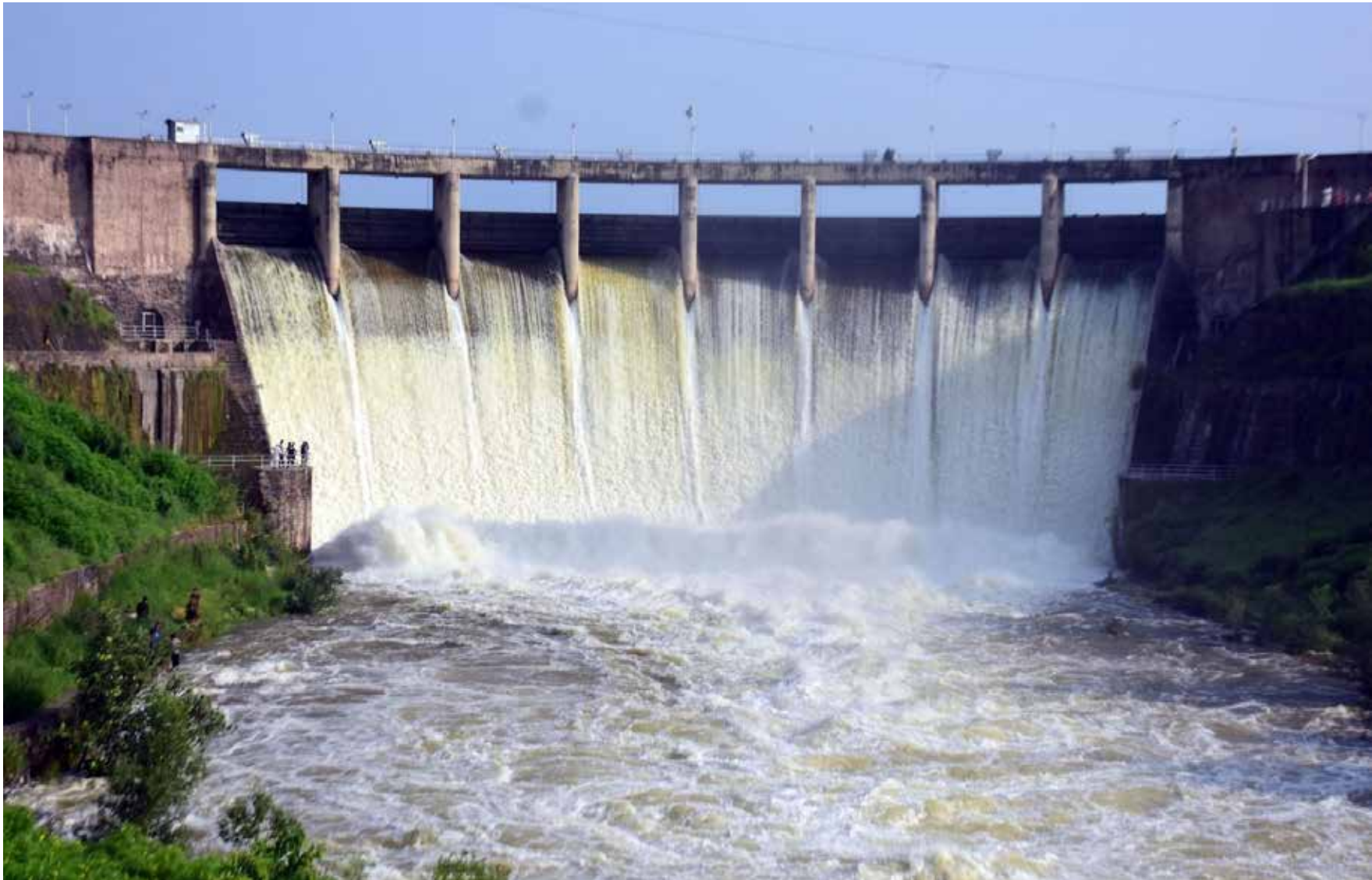
ISLAMABAD: District administration opened the spillways of Rawal Dam on August 25 at 6 am, and is actively monitoring the situation at rivers and bridges and has completed preparations for potential flood scenarios.— ONLINE
