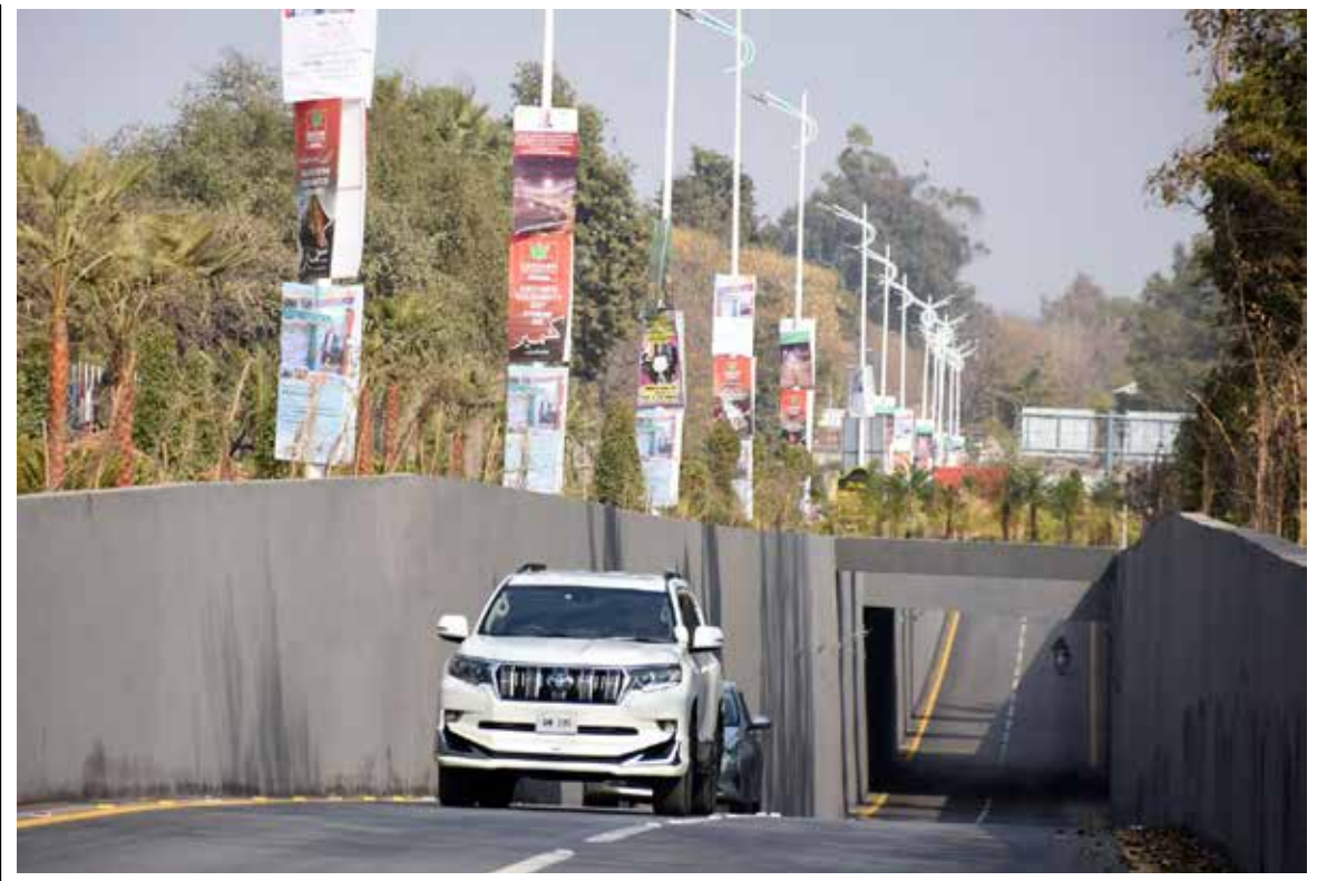
ISLAMABAD: Motorists are on their way through newly inaugurated Serena Interchange by Prime Minister, which is completed in record timing of 72 Days in Federal Capital
