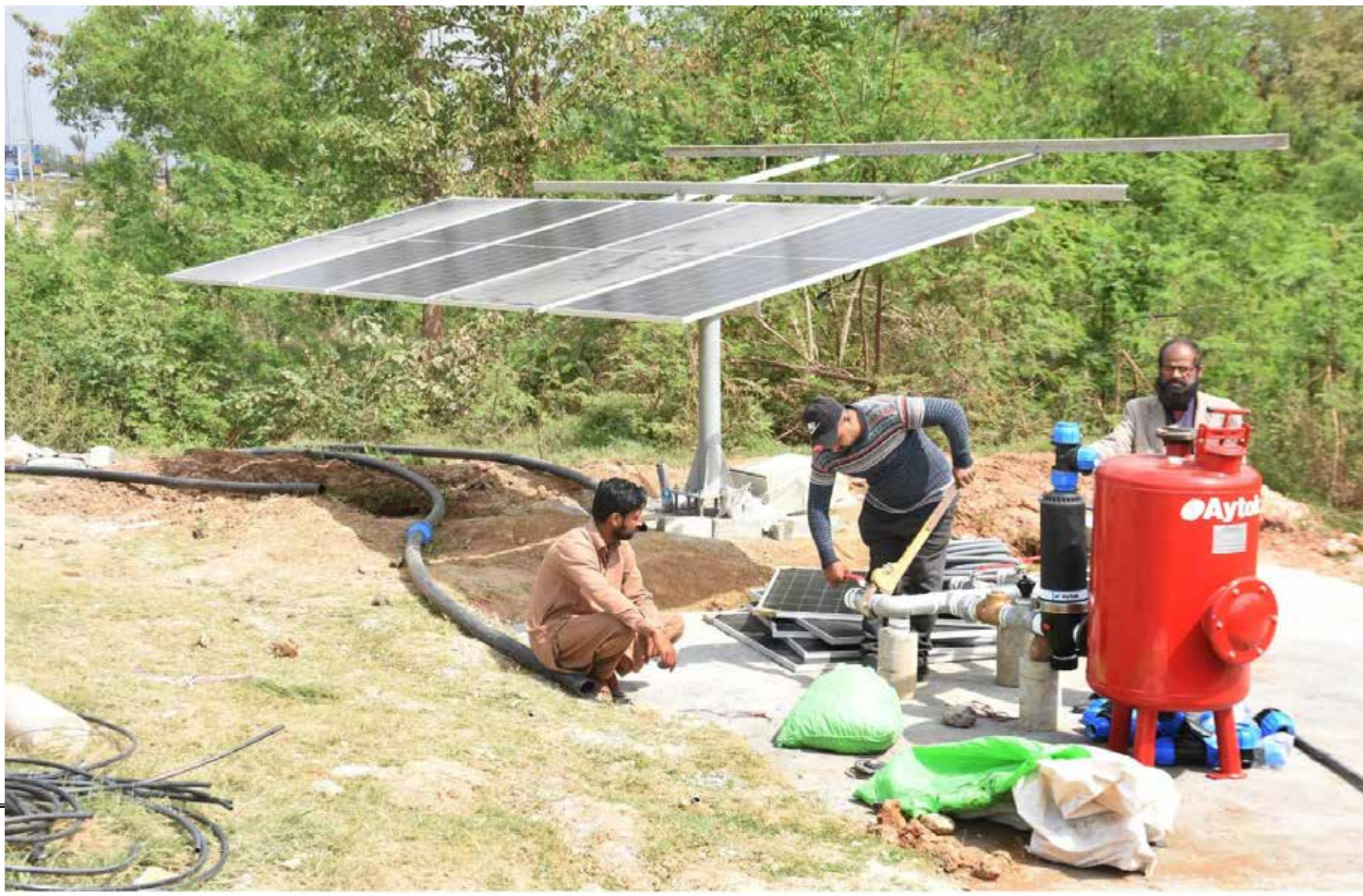
ISLAMABAD: Workers of local administration installing the setup for supplying the water to plants on green belts along the sides of Srinagar Highway as this new setup will run on the solar .
