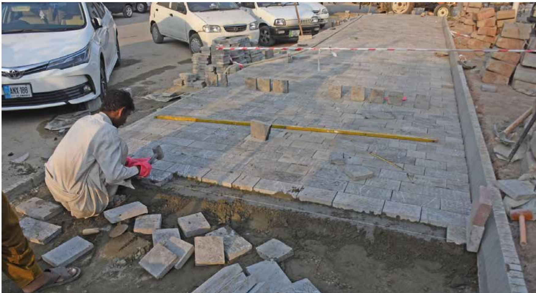
ISLAMABAD: Labourers busy in work at the Melody Food Park with a view to repair all damaged roads. – DNA
