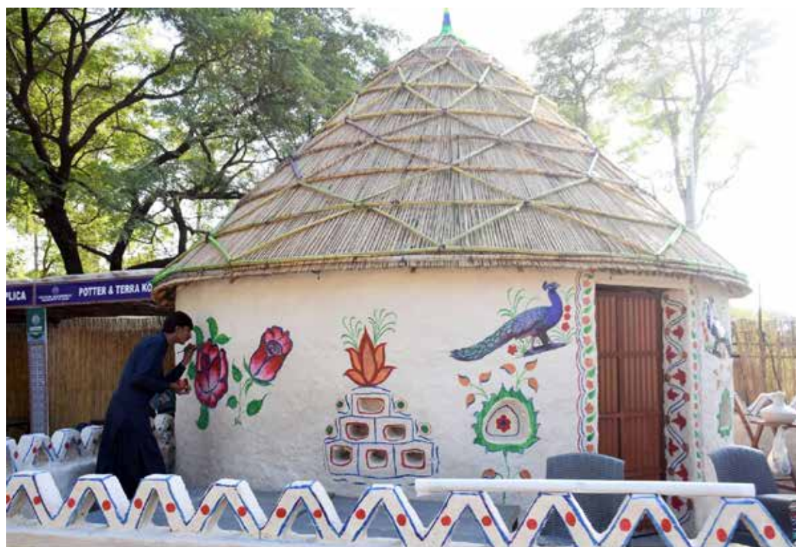
ISLAMABAD: Workers busy in final preparation for the different enclosures and pavilions at Lok Virsa.
