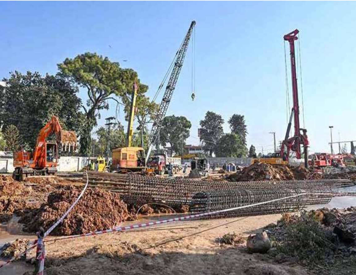
RAWALPINDI: Construction work underway on the major remodeling project of Kachehri Chowk, one of the busiest intersections linking Rawalpindi city, is underway to ensure a smoother traffic flow for over 200,000 vehicles passing daily through the twin cities' route.
