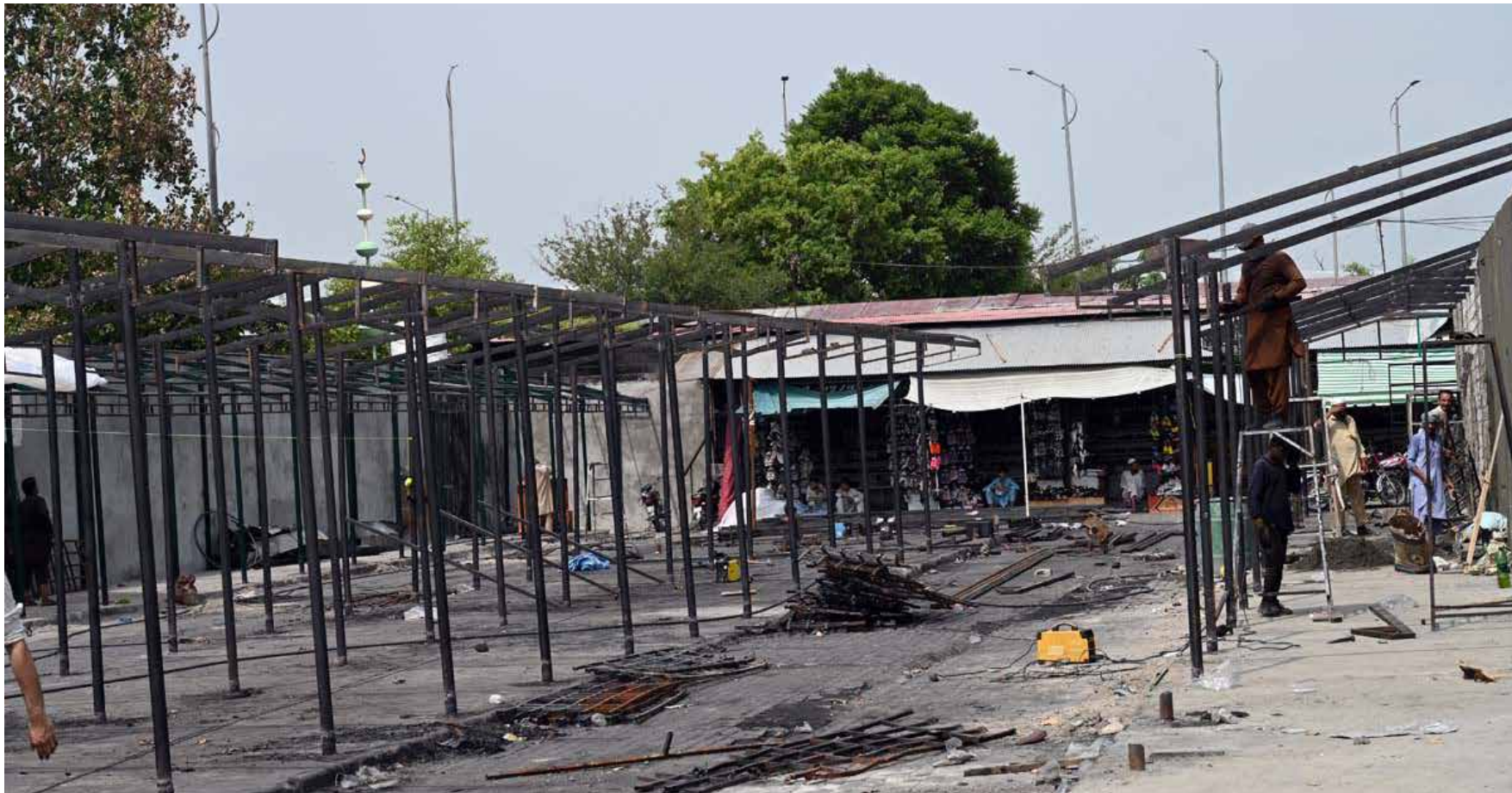
ISLAMABAD: Workers begin reconstruction and rebuilding of shops at H-9 weekly Bazaar.
